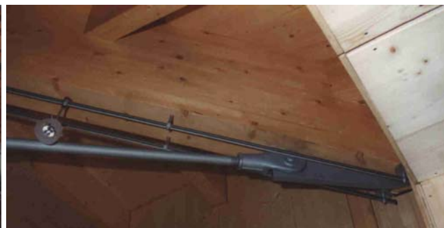
Gazebo roof structure
